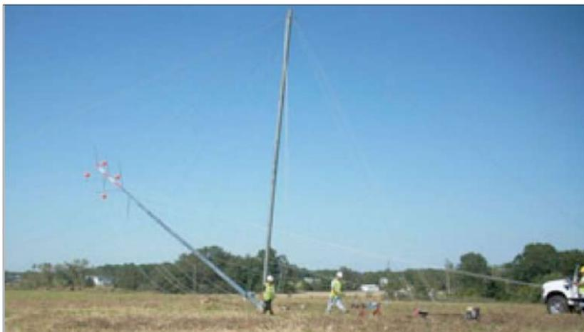
Photo courtesy Meskwaki Nation. The anemometer, used to measure wind force and speed, was installed on the meteorological tower last summer. Wind speeds will be gathered for a year before a decision is made to erect a wind turbine.
